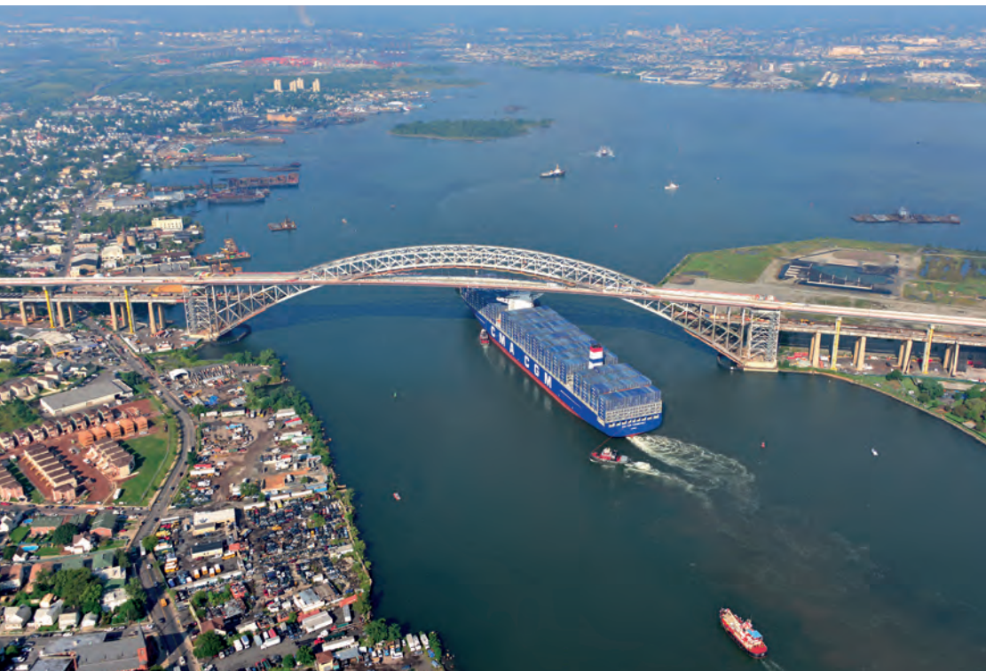
Bayonne Bridge, New Jersey/New York, USA
