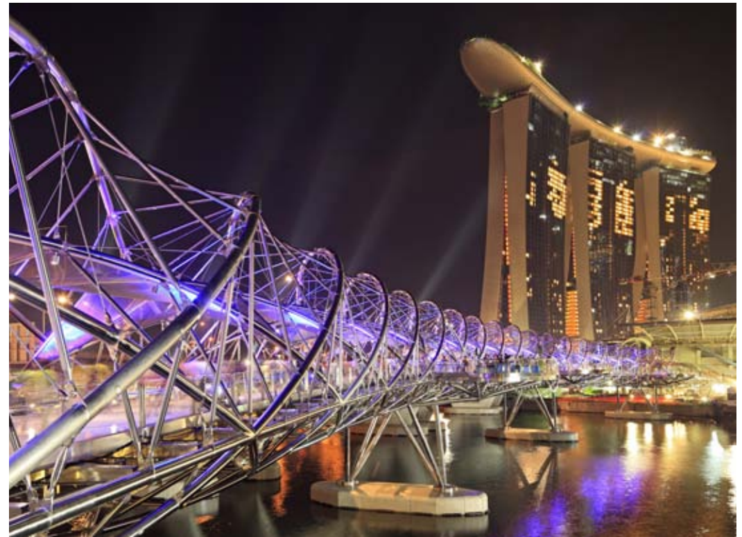
Marina Bay Bridge, Singapore. ©Darren Soh
