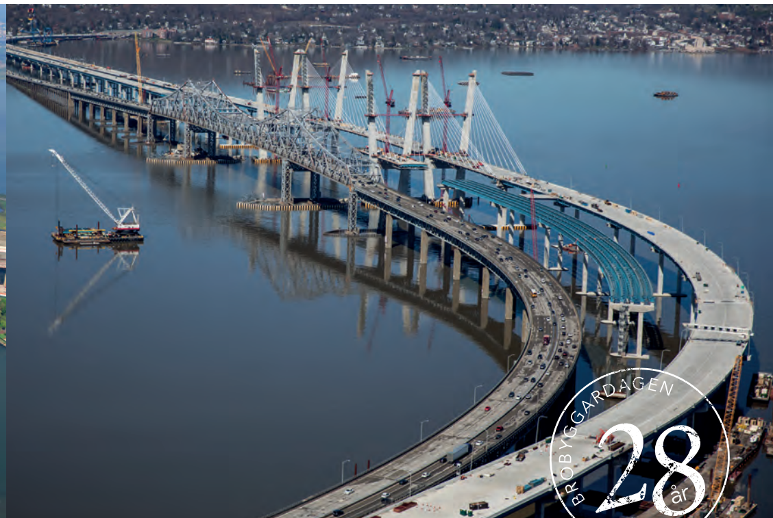
Governor Mario M. Cuomo Bridge, New York, USA
